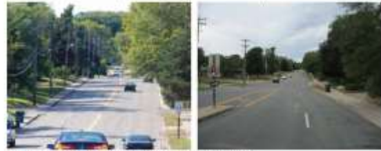
680 Street and Bryant, City of Bloomington, before and after a diet improvement
