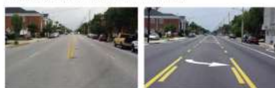
North 730th Street in Seattle, Washington, before and after a road diet improvement
